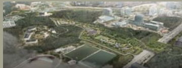
After construction of Bongnyeong Temple Citizens' Culture Park
